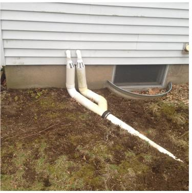
Sump Pump hard-piped to outside the house and connected directly into ground.
