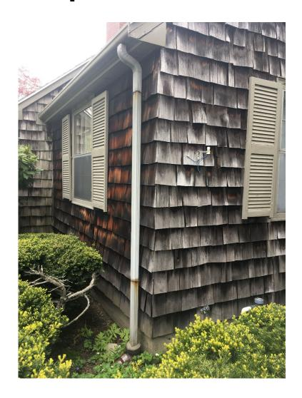
Roof Downspouts connected directly into ground, with unknown discharge location.
