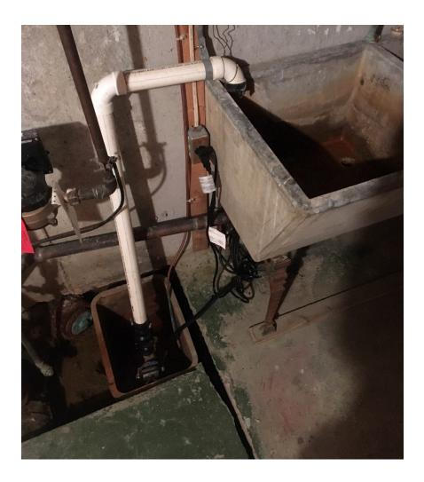
Sump Pump discharges to basement sink
