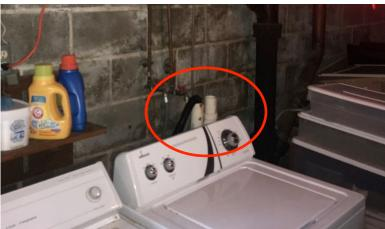
Sump Pump with flexible hose nearby to sewer connection (laundry machine drain pipe).
