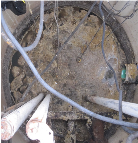
Normal grease buildup
