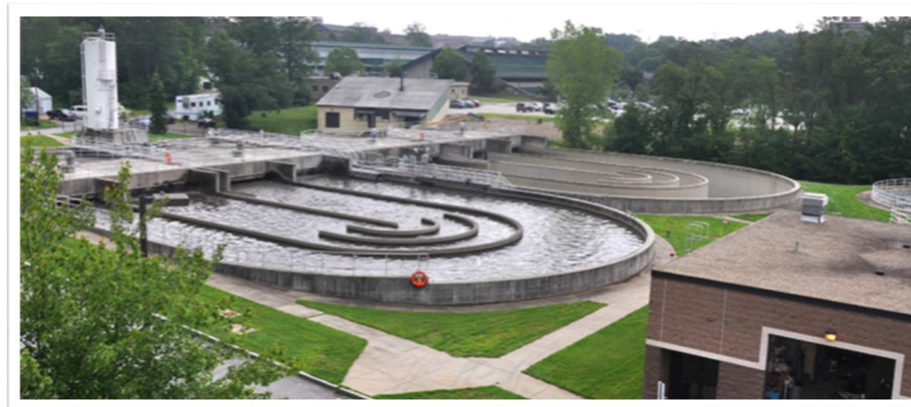
3.0 MGD Secondary Wastewater Treatment Facility
