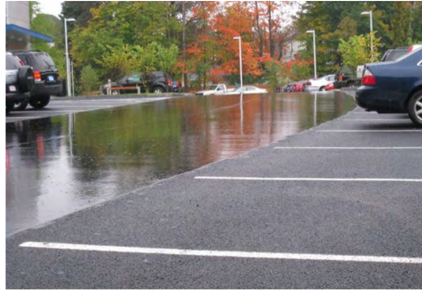
Porous asphalt in commercial parking stalls
