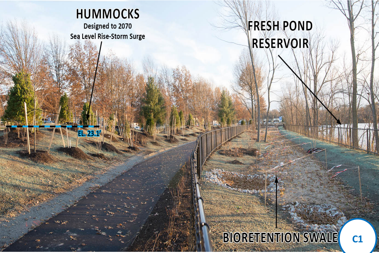
Build a vegetated berm at elevation 23.1 ft-CCB ( Cambridge city-based datum ) along Fresh Pond. This strategy could protect the Fresh Pond Reservoir for the projected 2070 100 year sea level rise / storm surge flooding.
