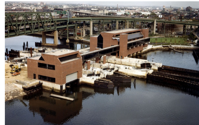
Charles River Dam (Source: New England District, US Army Corps of Engineers, 2015)
