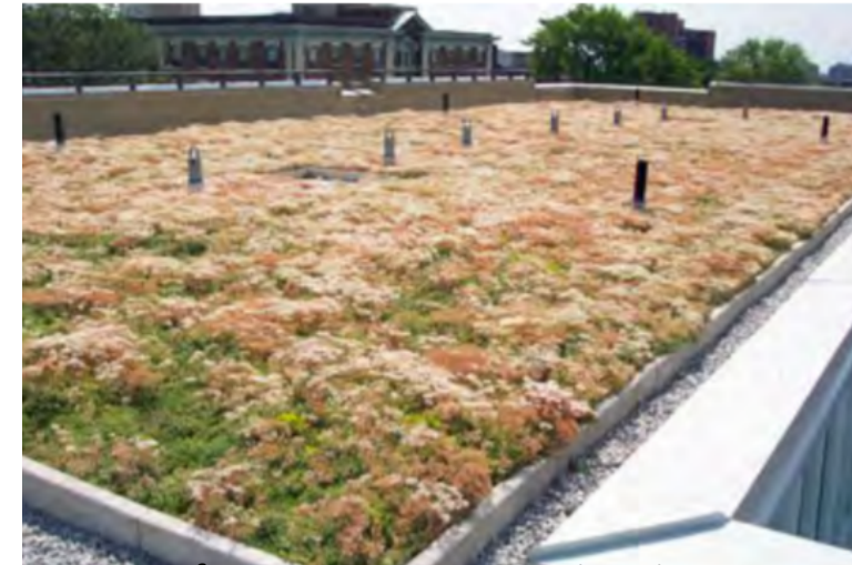
Green roof system at Ryerson University [Source: Toronto.ca – Green Roofs]
