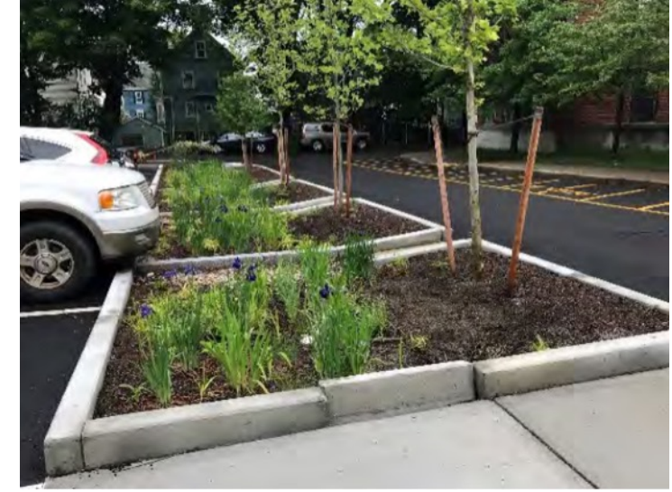
Tree planters and bioretention basin at parking lot of Irving School in Roslindale, Boston. [Source: BWSC and Greenovate City of Boston]
