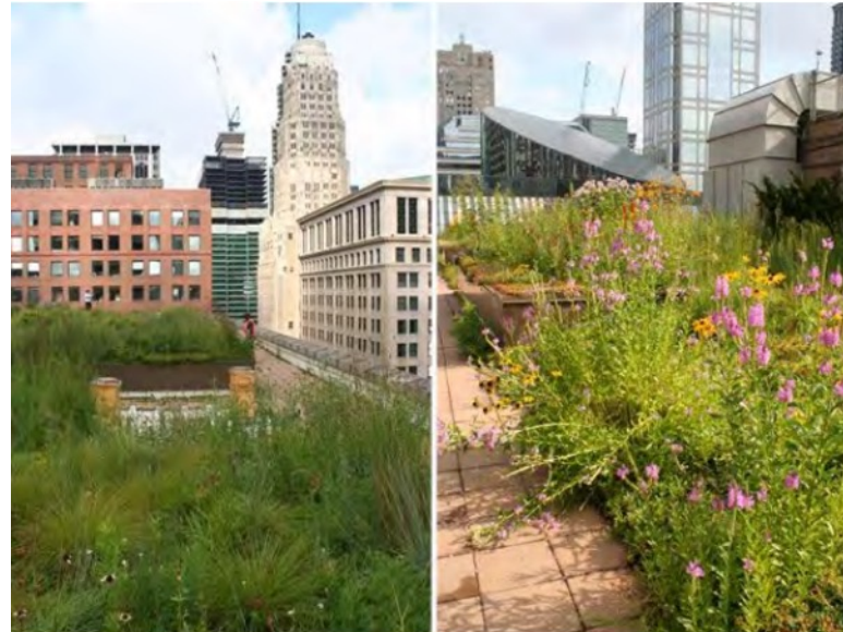
Chicago Green Roof. Photo credit: Conservation Design Forum
