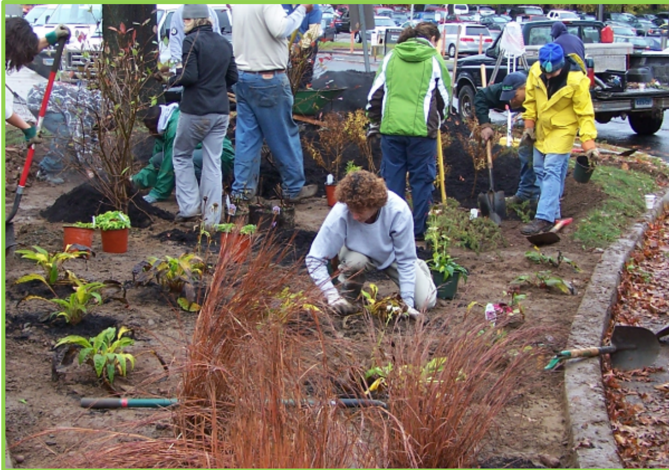
Rain garden installation Hartford, CT
