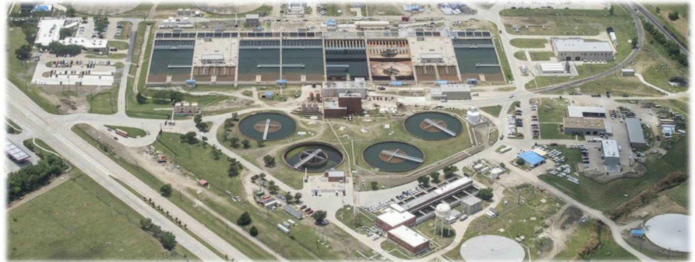
800 MGD NTMWD Wylie Treatment Facility
