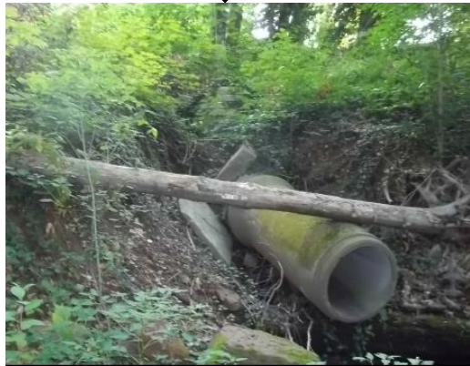
Elmwood Avenue outfall
