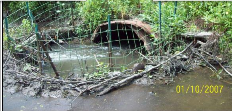
Pondside Road culvert inlet south of Birnie Road
