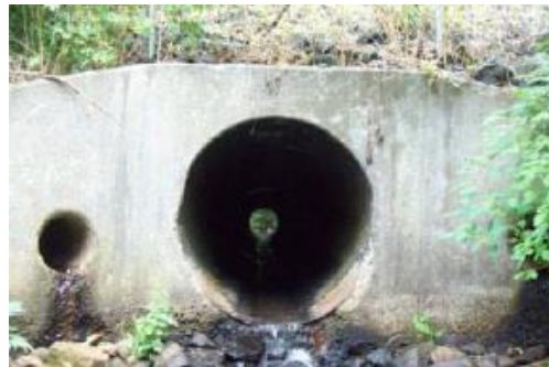
Mill Brook Culvert at Mill Road
