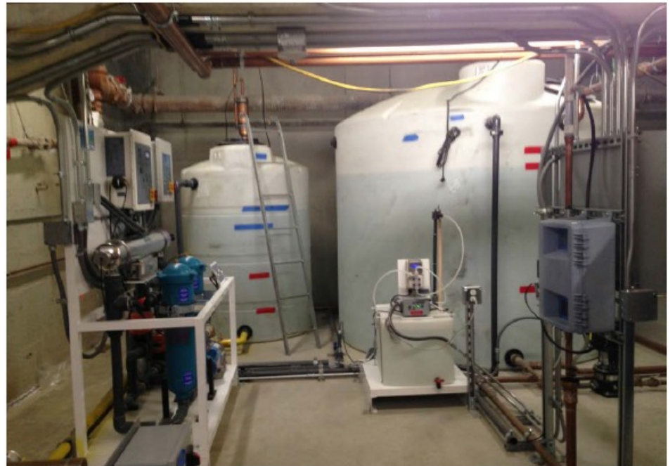
2270 Folsom Street's non-potable water reuse system
