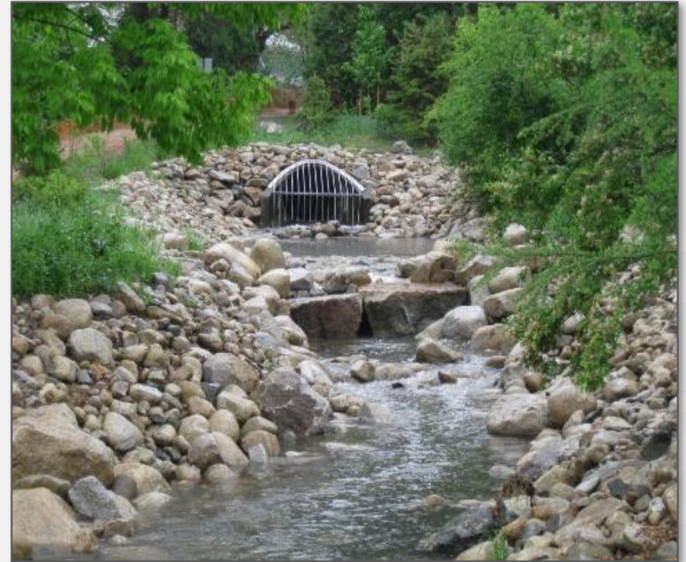
Outfall Reconstruction & Permanent Erosion Control
