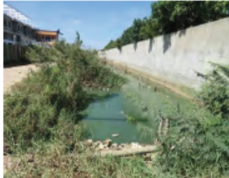
Existing Drainage Channel (2/2)
