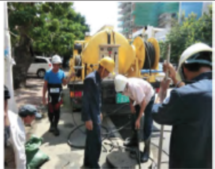
Pipe Cleaning by DSD
