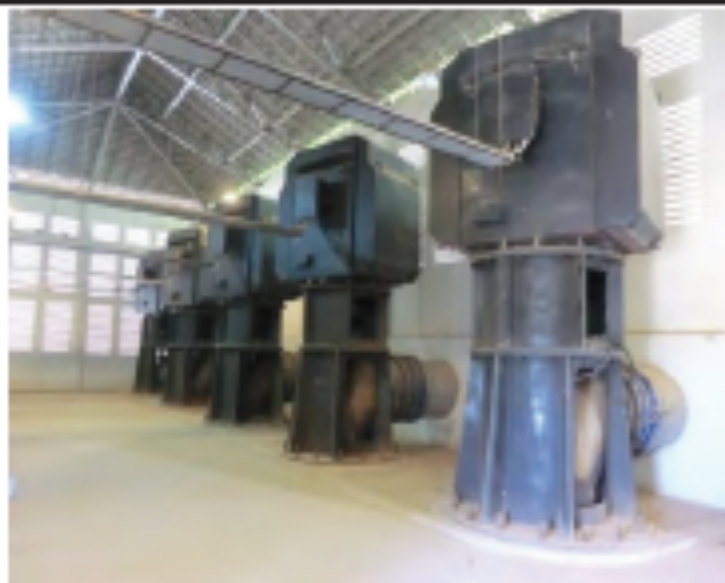
Existing Pumping Station (Kop Srov Pumping Station)
