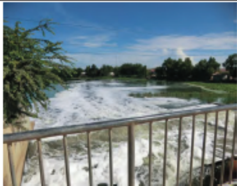
Discharged Water from Kop Srov Pumping Station
