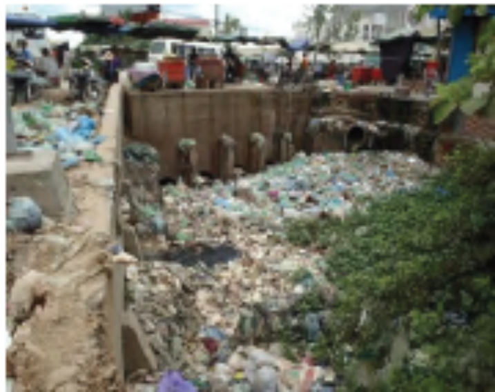
Existing Drainage Channel (1/2)
