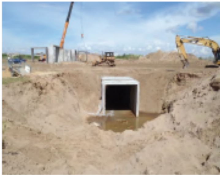
Box Culvert in Development Area (Under Construction)
