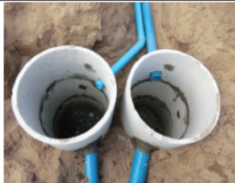
Septic Tank (Under Construction)
