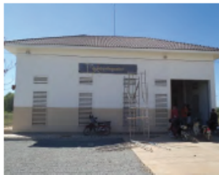
Existing Pumping Station (Tuol Sampeo Pumping Station)
