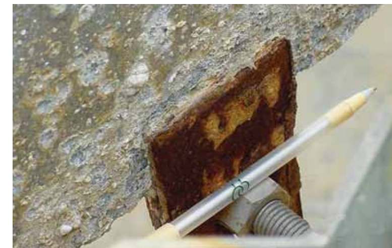
Figure 2. Close-up of aluminum clarifier baffle—electrically continuous with carbon steel rebar in concrete
