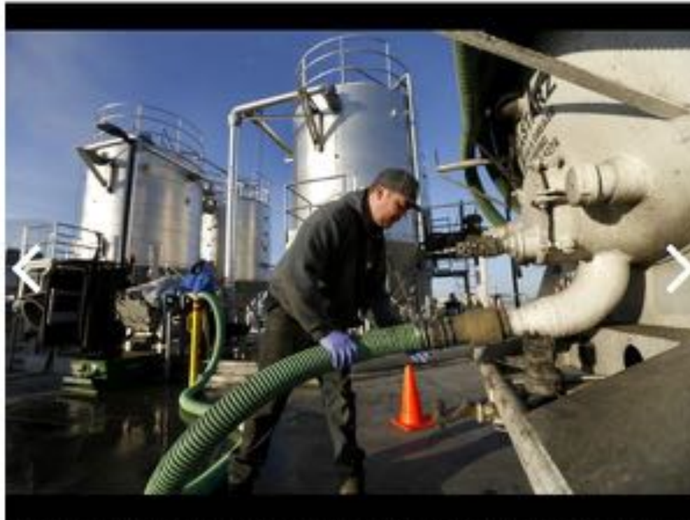
(1 of 2) Ken Kolp of North Bay Restaurant Services hooks up a hose to transfer septic tank sludge from his truck to a high strength waste system at the Laguna Treatment Plant in Santa Rosa, on Tuesday, December 20, 2016. (BETH SCHLANZER/The Press Democrat)
