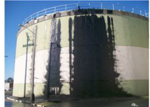
Sludge escaping from the fixed cover digesters in Nashville
