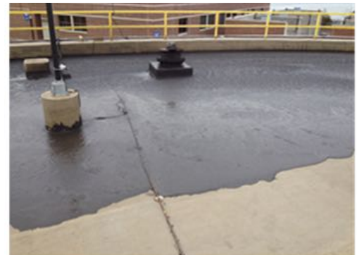
Sludge on the covers of Hunts Point digesters
