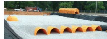
Typical installation of underground infiltration system below an existing parking lot.
