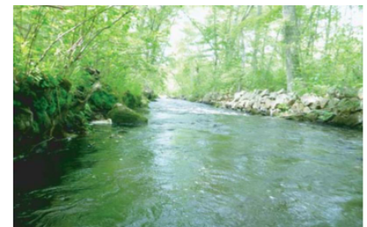
Granite-lined, straightened mill-race channel with restricted floodplain access, located downstream of Route 112.
