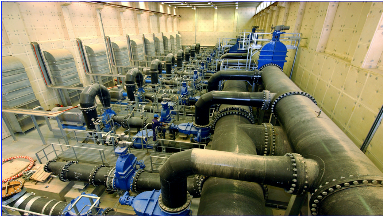
Fig. 1. Main pumping station
