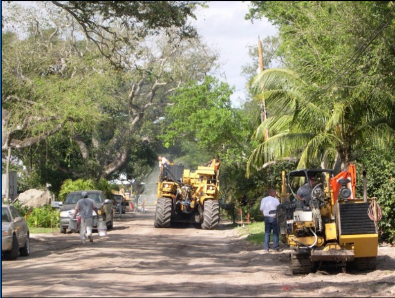
Construction of Gravity Sewer Mains
