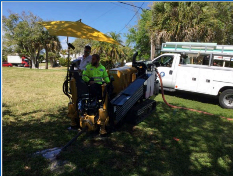
Directional Drilling of STEP Sewer Mains
