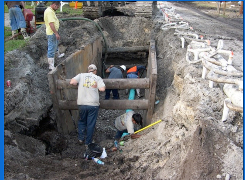
Open Trench Excavation of Gravity Sewer Mains
