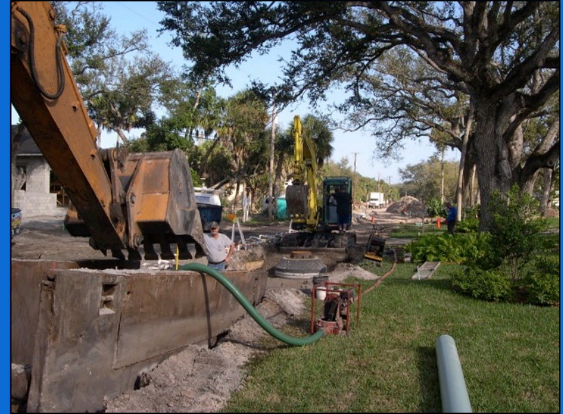
Dewatering of Open Trench for Gravity Sewer Installation
