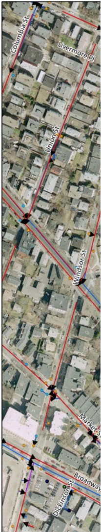
Webster Ave Sewer Infrastructure
