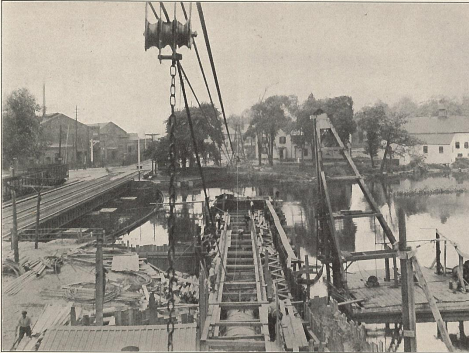
OUTFALL SEWER—FIRST SECTION OF COMPLETED COFFERDAM
