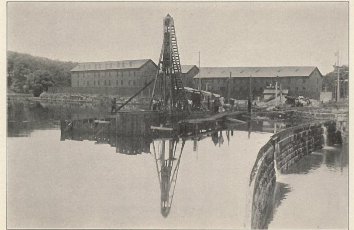
OUTFALL SEWER—DRIVING STEEL PILES FOR COFFERDAM
