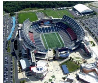
250,000 GPD on-site water reuse system for New England Patriots, Foxboro, MA
