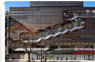
The New School University, NYC 40,000 GPD in-building onsite water treatment & reuse for flushwater, cooling, irrigation & laundry.
