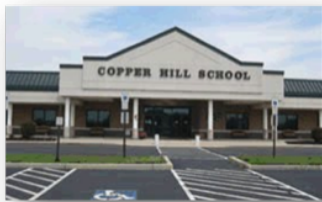
Copper Hill Elementary School, East Amwell, NJ 1 st public school water reuse system
