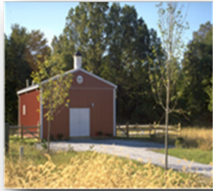
Small Community On-site Wastewater Treatment 40 homes; Agriculture/ Open Space Preservation.
