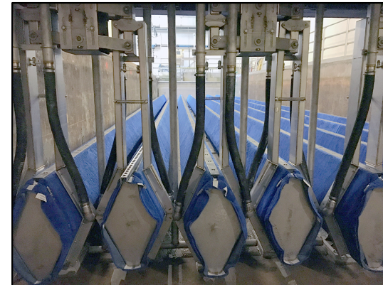
Five of eight diamond laterals at influent end of tank
