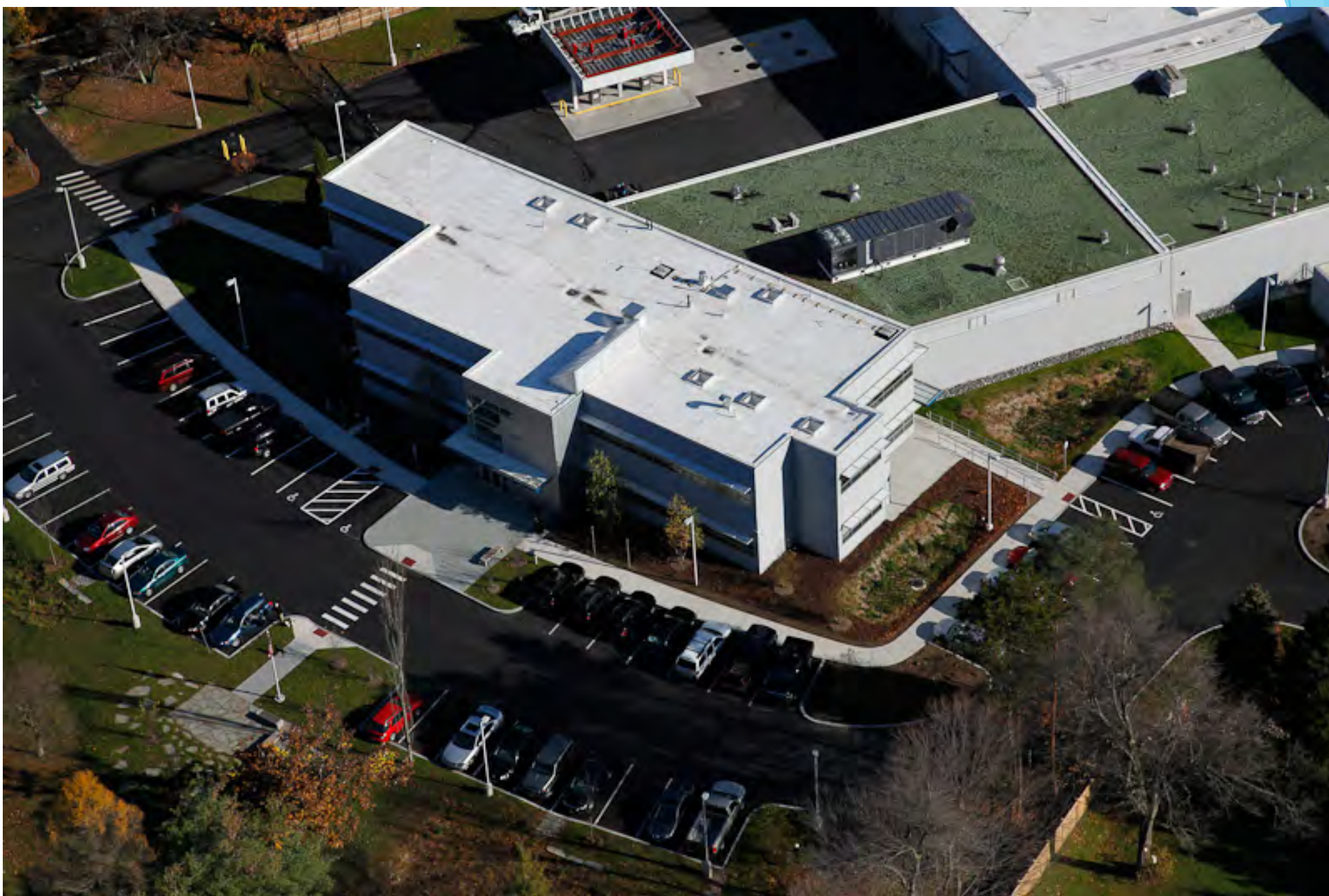
Public Works Facility, Lexington, MA LEED Silver Certified
