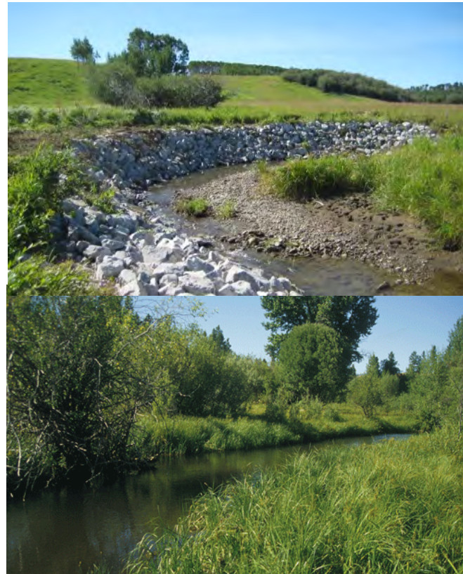
Riprap or Bioengineered Bank
