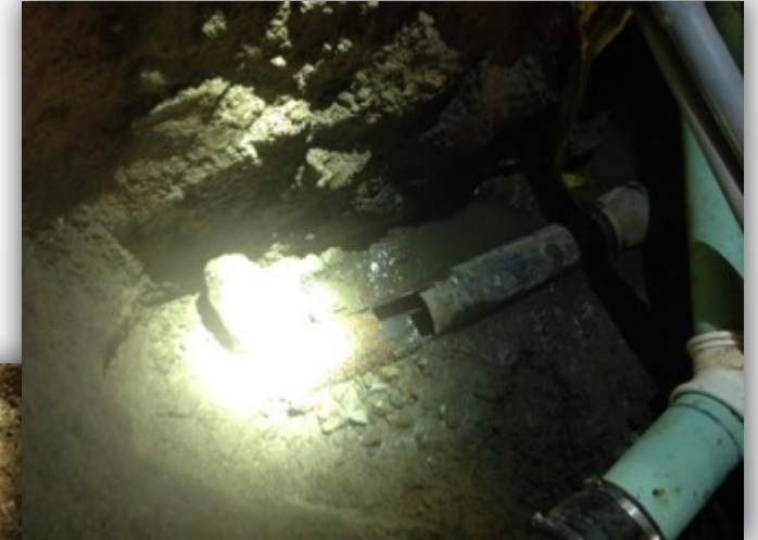
A sewer line was found connected to a DMH on Main Street
