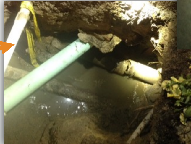
A sewer line was found connected to a DMH on Main Street
