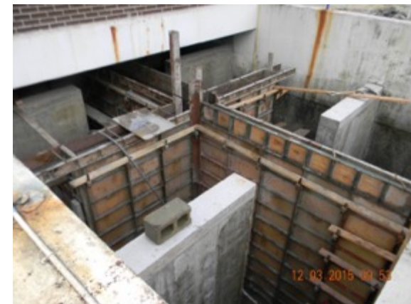
Chlorine Contact Tank Rehabilitation
