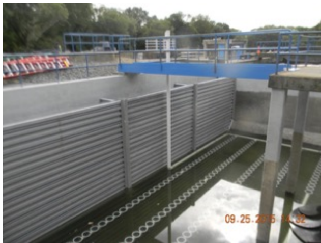
New Diffused Aeration
