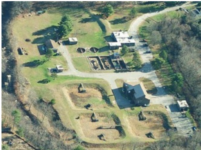
North Plant – Design Flow = 1.086 MGD
