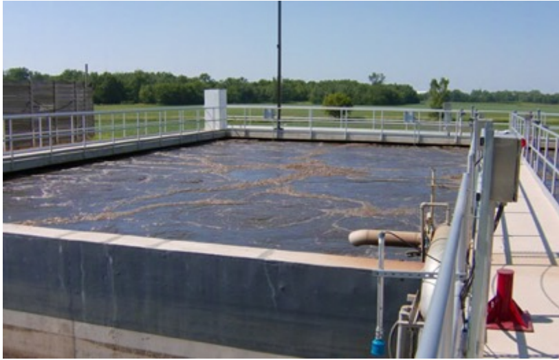
Sequential Batch Reactor
