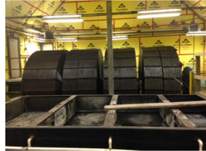
Rotating Biological Contactor
