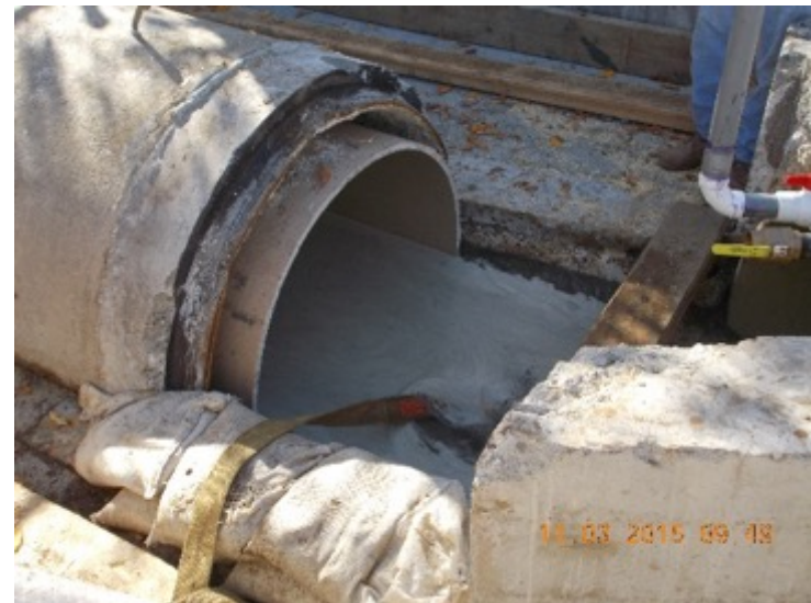
Grout Leakage into Pipe
