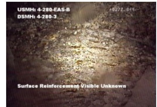
Loss of concrete and exposed reinforcement were observed
