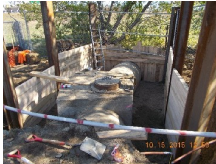
Access Opening Construction
