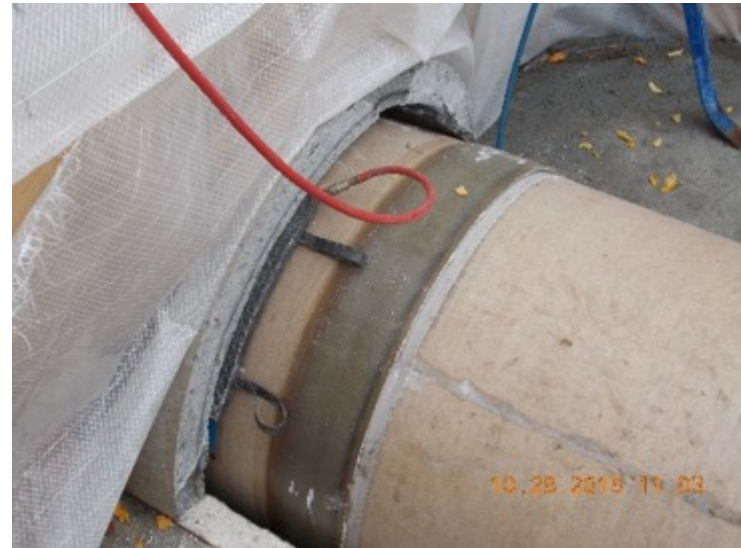
Pipe Installation – Pipe held in place for joining
