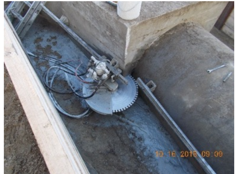
Concrete Cutting at Manhole
