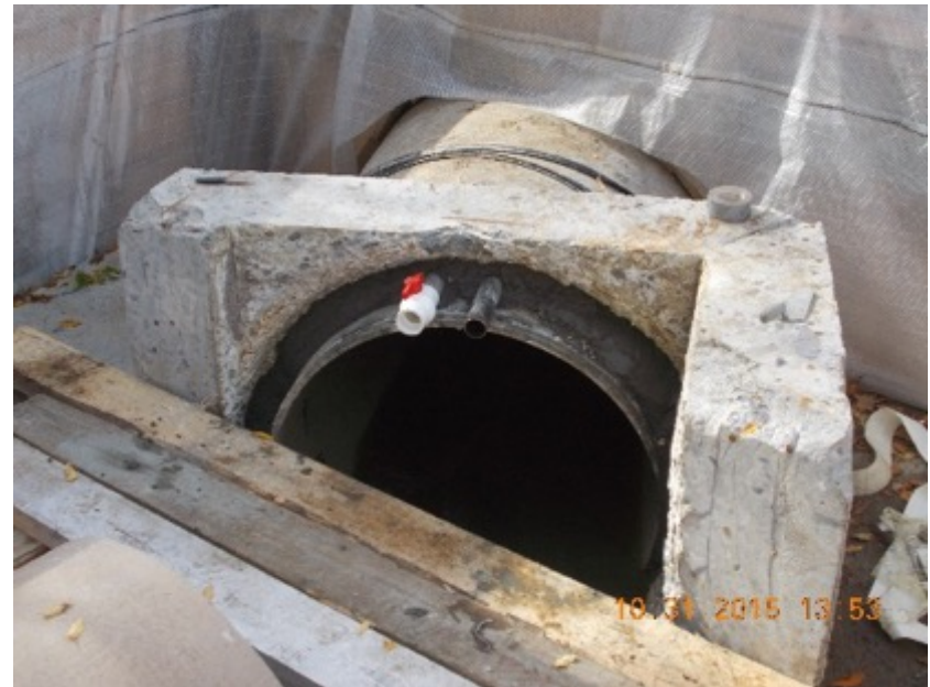
Bulkhead with Grout Port and Air Release Lines
