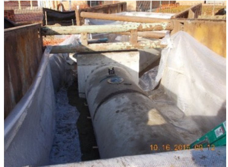
Flow Containment Controls
