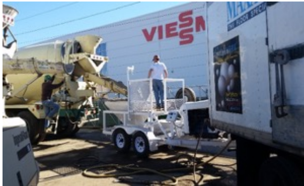
Grout Pump and Foaming Agent Truck
