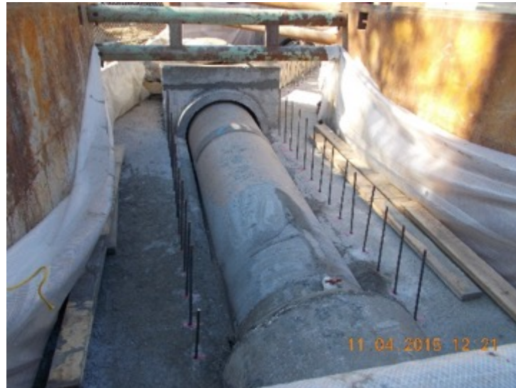
Rebar for Concrete Encasement
