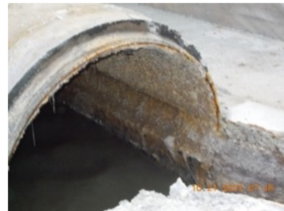
Existing Sewer exposed during construction
