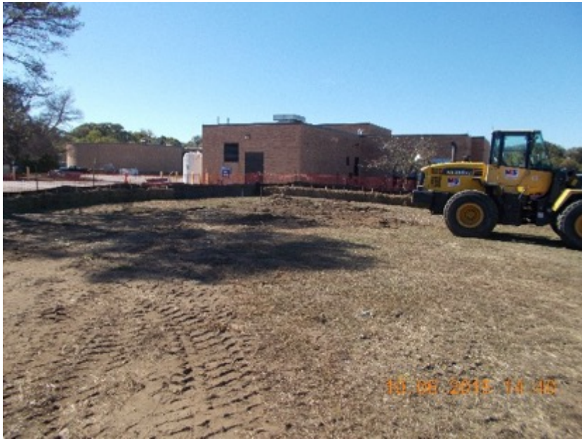
Staging and Laydown Area
