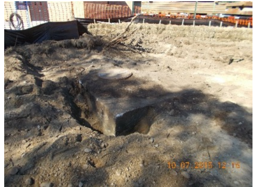
Exposing Existing Sewer
