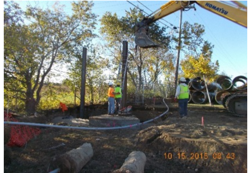
WSA fence removed – RIDOT fence intact
