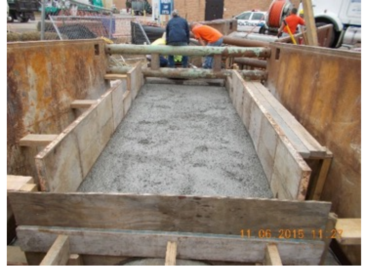
Completed Concrete Encasement
