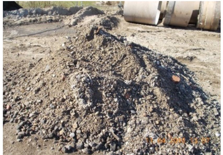
Debris Removed from Screen Chamber in Headworks
