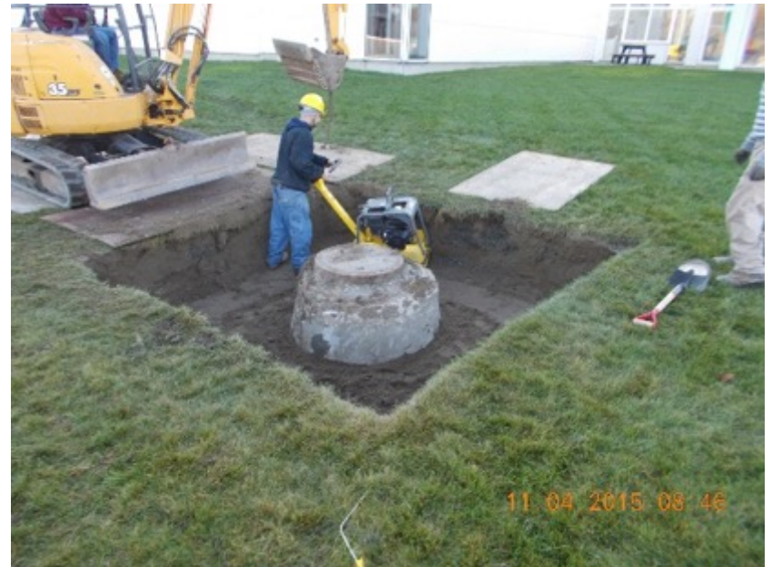
Sliplining Receiving Location Restoration
