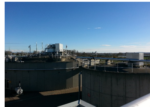
Lulu Island, Vancouver, BC digesters lithium study showed 100% active volume in the digester
