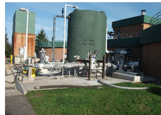
Gresham, OR FOG receiving station is used to enhance biogas production for renewable energy production.
