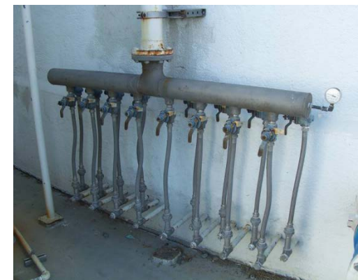
Gas piping for digester mixing
