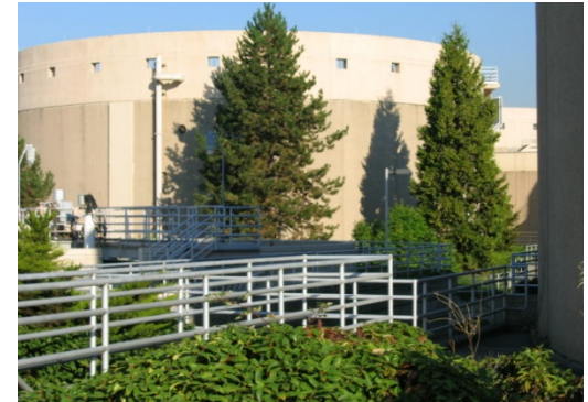
King County mesophilic anaerobic digesters mixed with a combination of pumps and gas spargers
