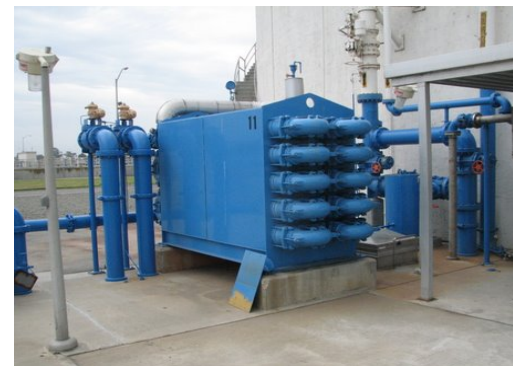
Tuning heat exchanger at San Jose
