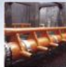
Air Distribution System — Oklahoma City, Oklahoma, OK. Uniform air distribution system provides even airflow across the reactor with 1-4% waste concentration or more.
