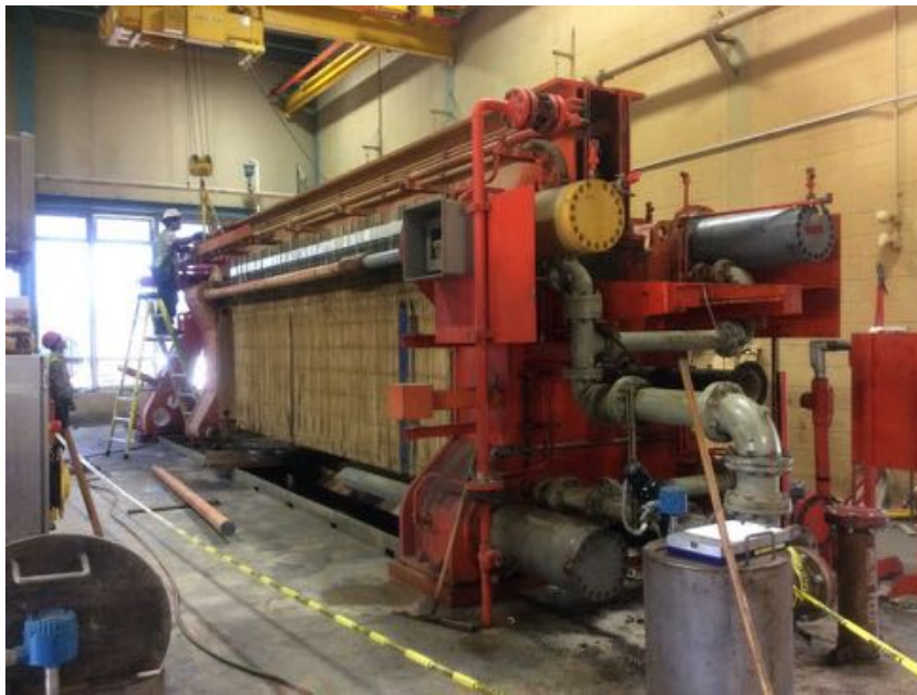
Old Plate and Frame Presses with Lime Stabilization
