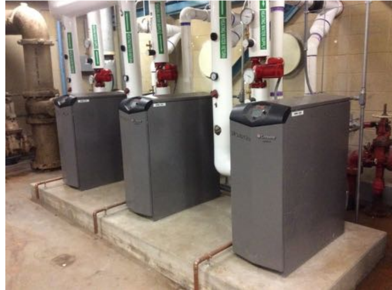
New Propane Hot Water Boilers
