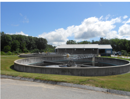
Two AMWELL Stainless Steel Circular Secondary Clarifiers
