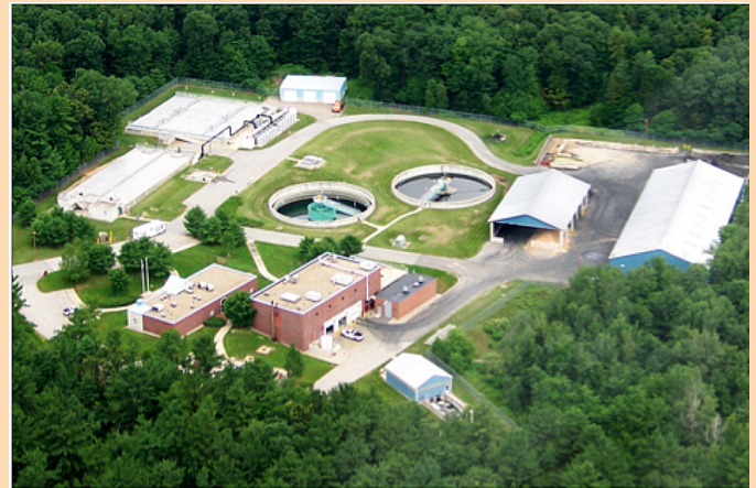
Dover, NH WWTF
