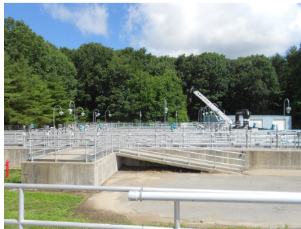
MLE Process with Invent Mixers and Aquarius Technologies Aeration System
