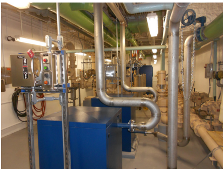
Four new Aerzen Channel and Septage Blowers and Two new Carter Plunger Pumps
