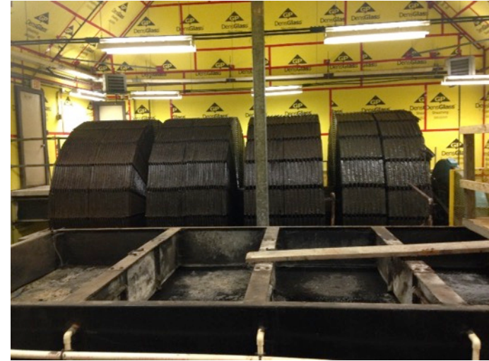
Rotating Biological Contactor
