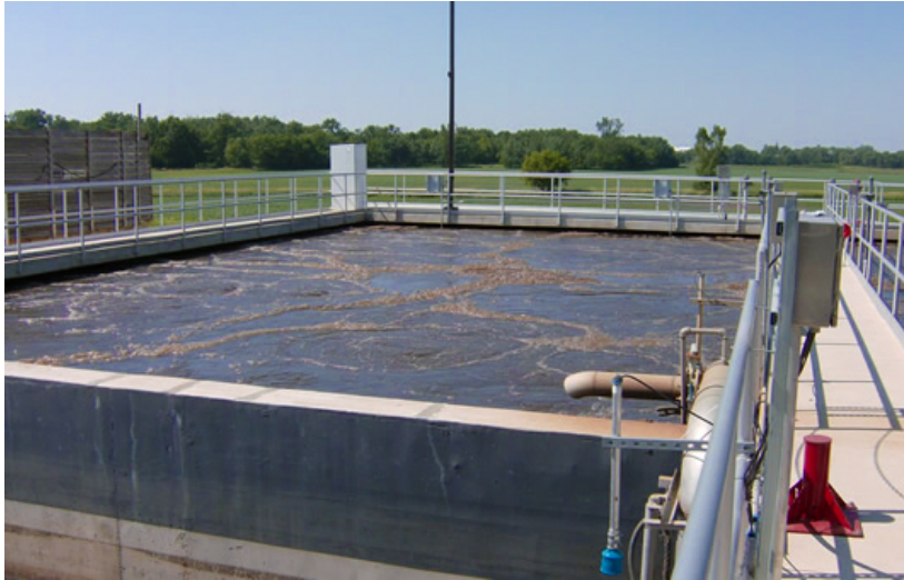
Sequential Batch Reactor
