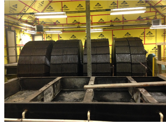
Rotating Biological Contactor
