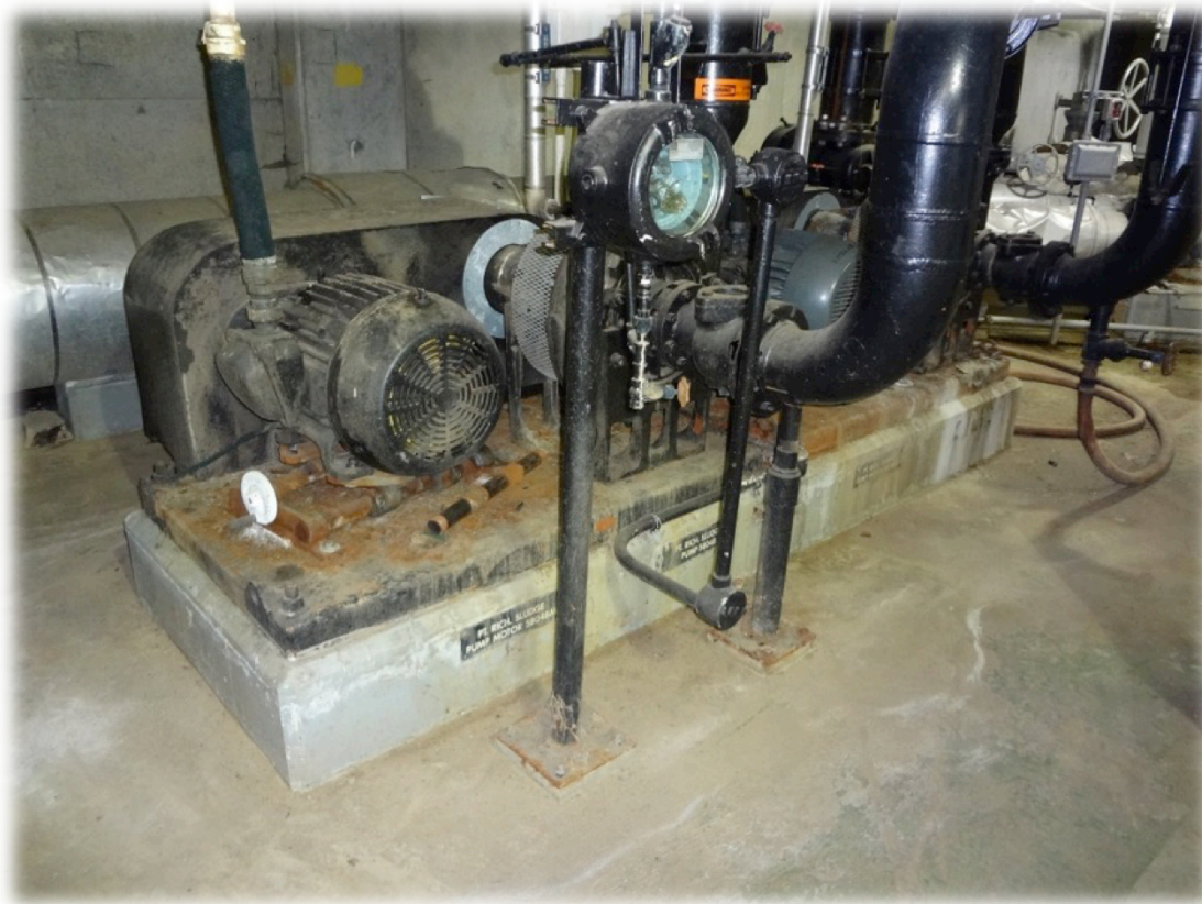
Digester Sludge Transfer Pumps
