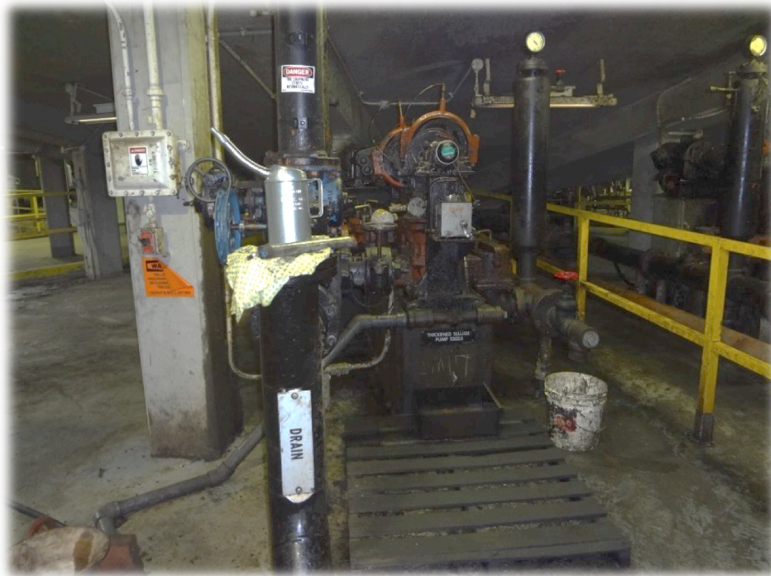
Thickened Sludge Pumps (Replace with Progressing Cavity)
