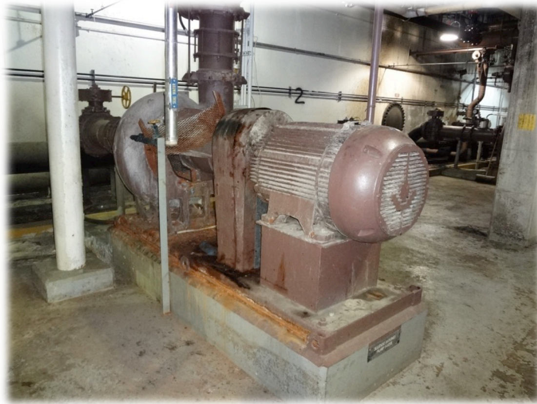
Digester Sludge Mixing Pumps
