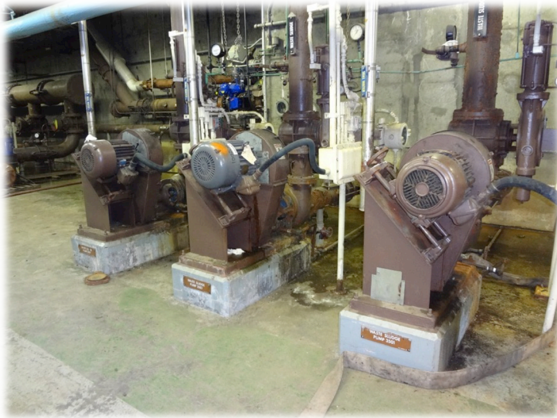
Waste Activated Sludge Pumps (Replace with Progressing Cavity)
