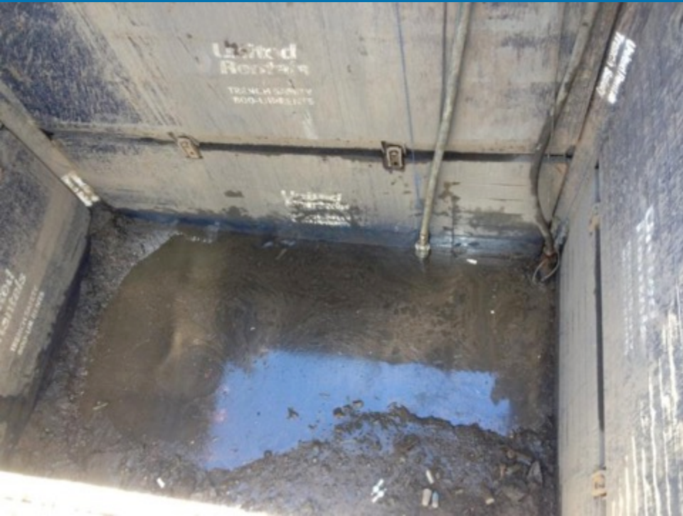
Excavation Support System
