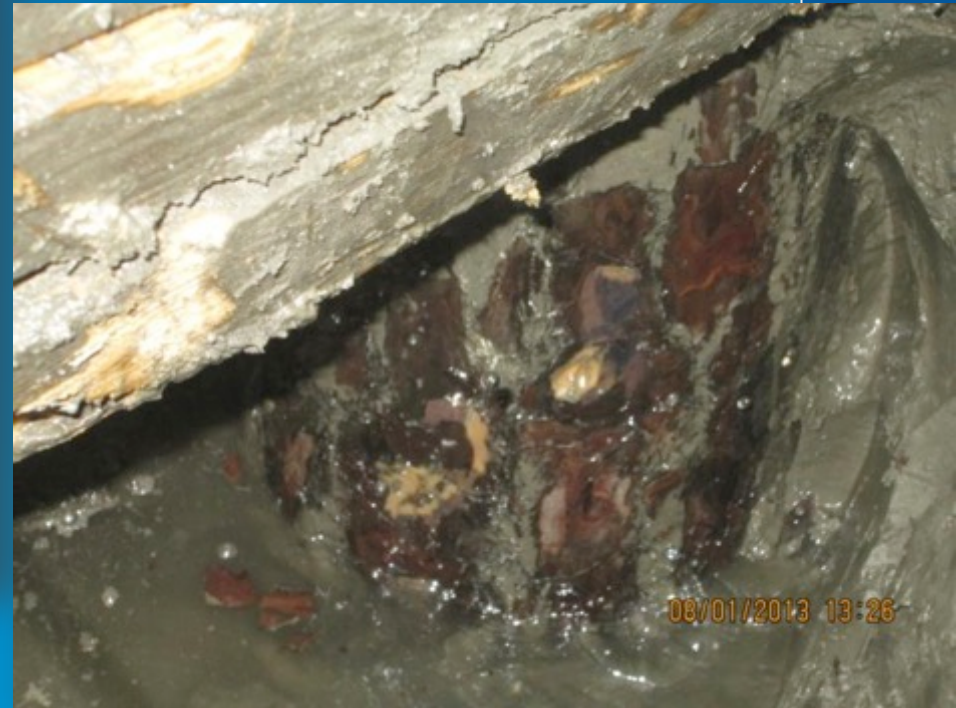
Exposed Timber Pile Cap and Pile
