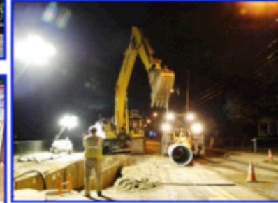
East Framingham Sewer Improvement Project
