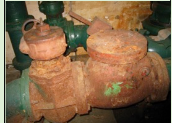
Deteriorated Pump Station Equipment
