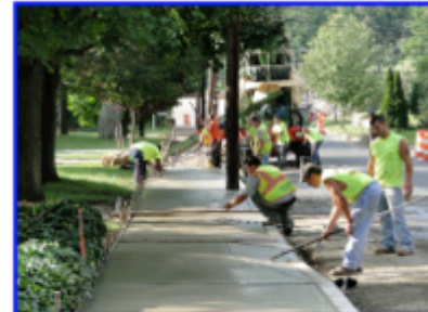
State Street Roadway Reconstruction Project
