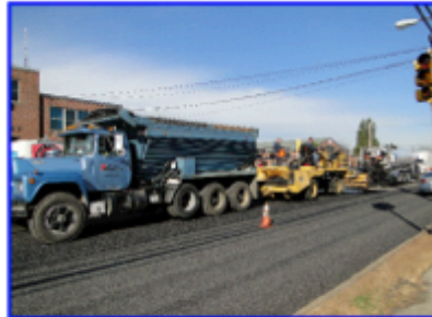
South Concord Street Roadway Reconstruction Project
