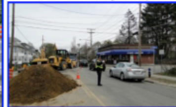
Grove and Peab Street Sewer Main Replacement Project
