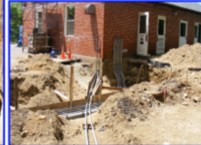
Pleasant Street & Grove Street Pump Station Replacement Project
