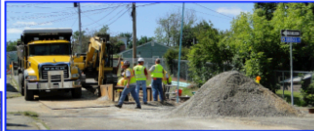
Cohasset Area Water Main and Sewer Main Replacement Project
