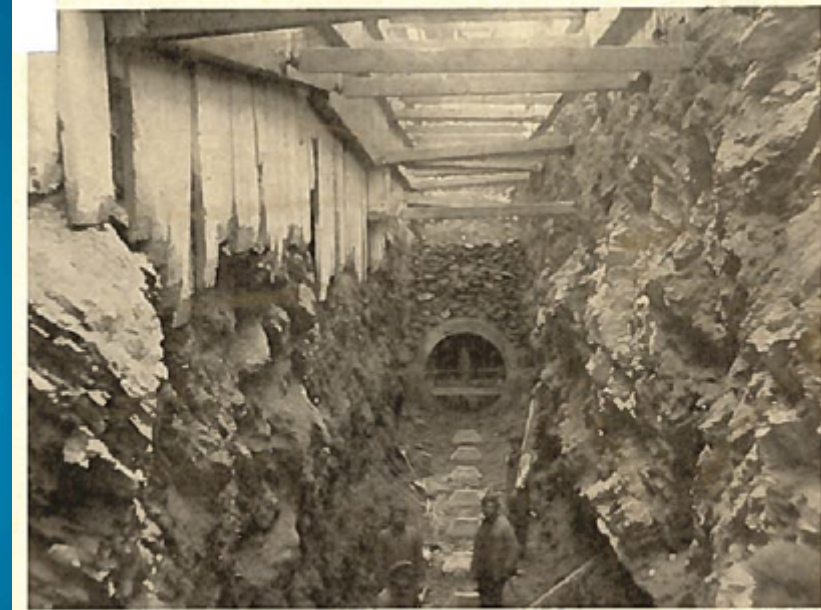
TWENTY-SIX FOOT ROCK EXCAVATION FOR SIX-FOOT CEMENT SEWER
