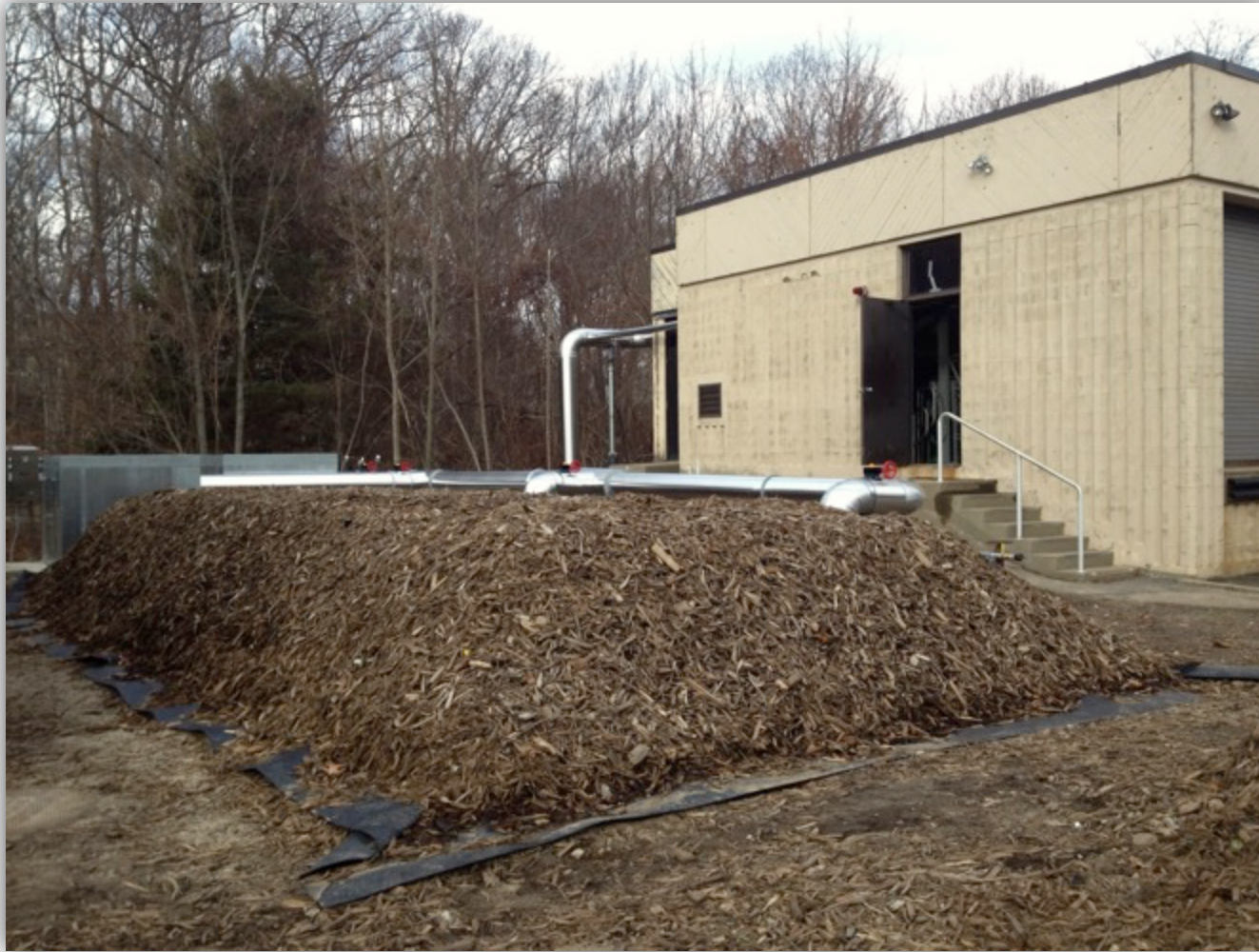
2012 Headworks Upgrade & Odor Control 900 cfm
