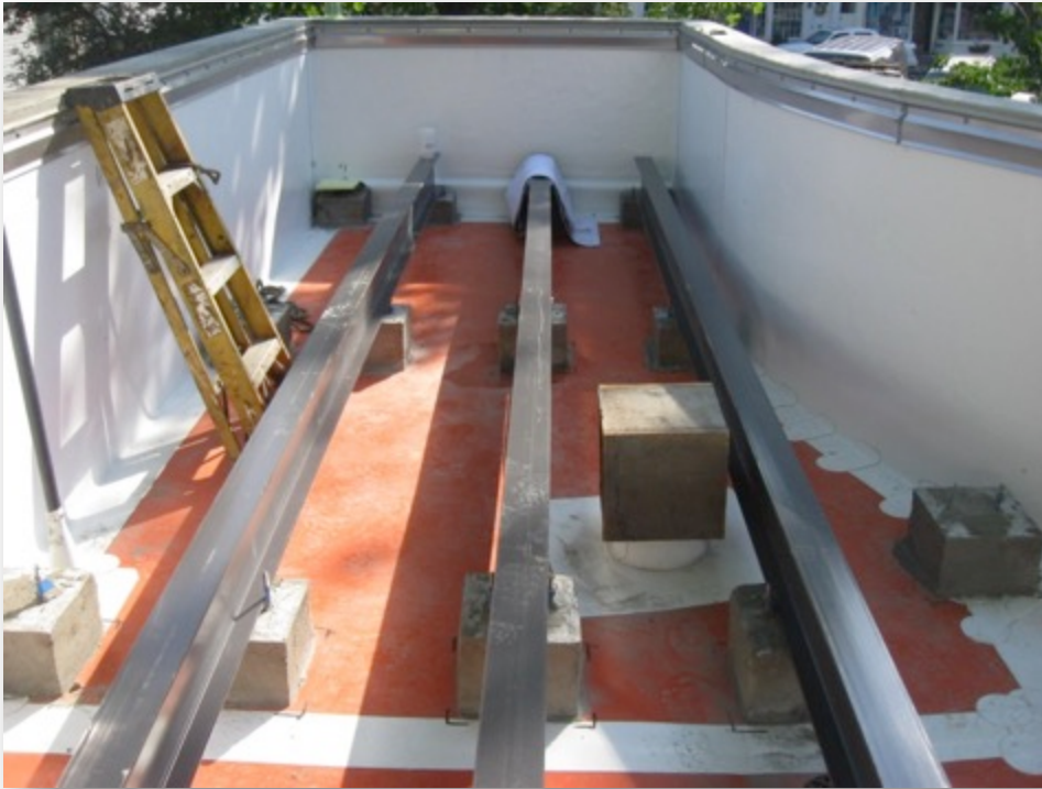
Media Support System: FRP Beams & FRP Grating
