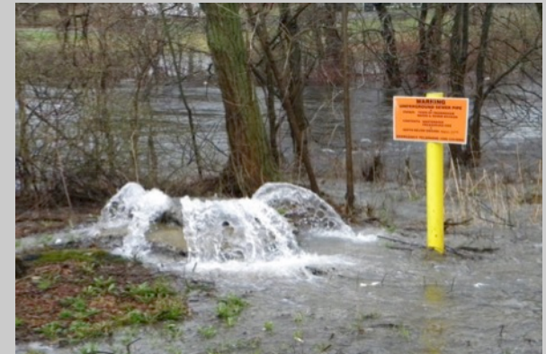
Sanitary Sewer Overflow March 2010
