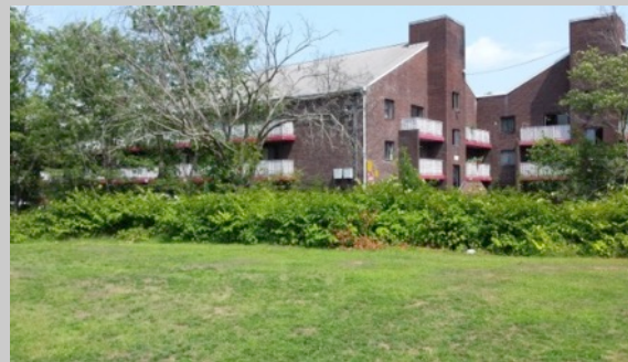
Looking east from park. Note: invasive Japanese knotweed dominating western bank
