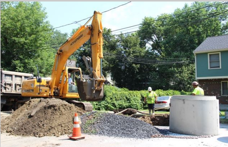
Installing drainage manholes May 2015
