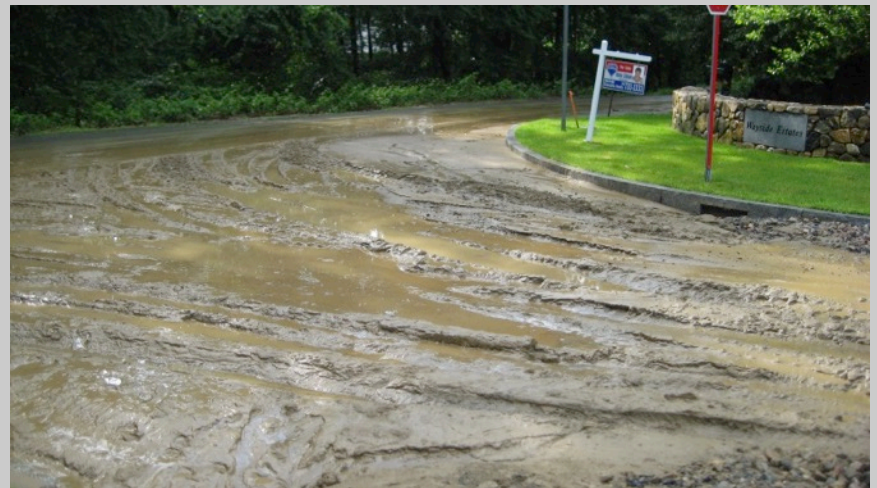
Construction site runoff July 2009
