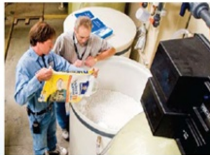
PHOTO: Boeing heating, ventilation and air-conditioning mechanic Brett Weberg adds salt used in regeneration tank for cooling-tower water softeners at the Kent, Wash., site. The water softener is part of a new process initiated by lead mechanical engineer Roger Sampair (right) that will save water and reduce sewage and maintenance costs across Boeing. MARINA LOCKHART/BOEING
