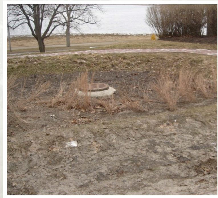
Clifton Street Sewer Separation Project Hersey Street - March 2011
