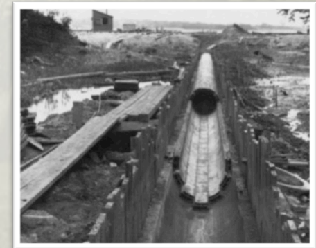
Portland Dartmouth Street Combined Sewer, 1918
