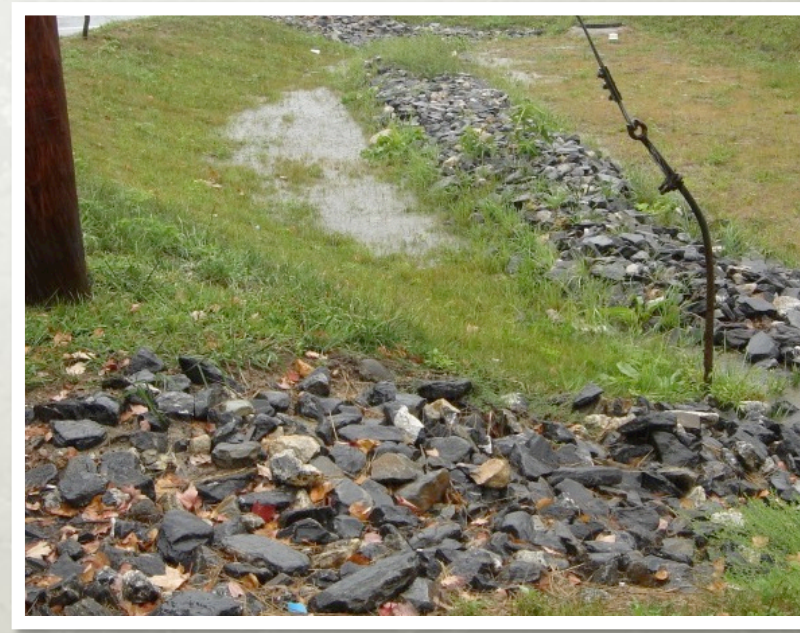
Read Street Sewer Separation 2008-2009
