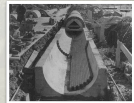
Portland West Side Interceptor, 1940
