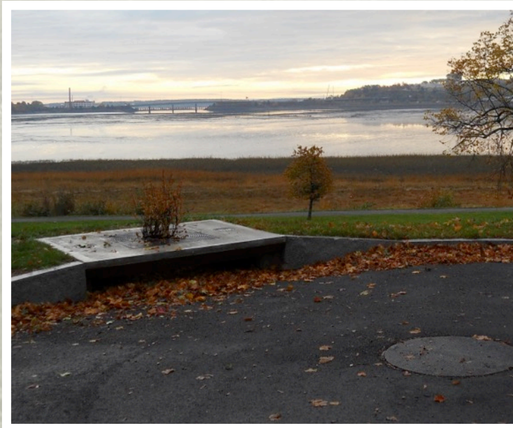
Mackworth & Austin Streets Clifton Street Sewer Separation 2009-2010
