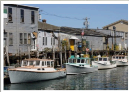
Portland viewed from the waterfront – Old Port District
