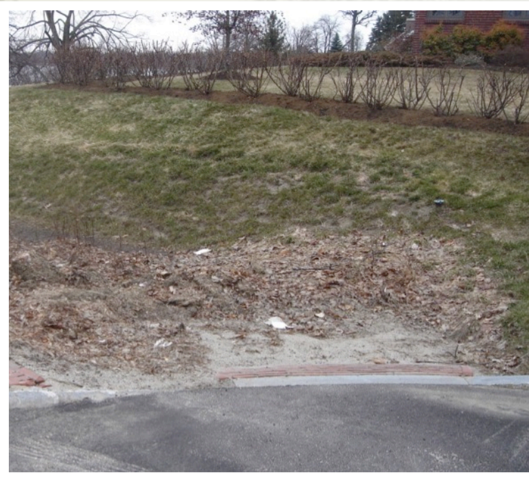
Clifton Street Sewer Separation Project George Street - March 2011
