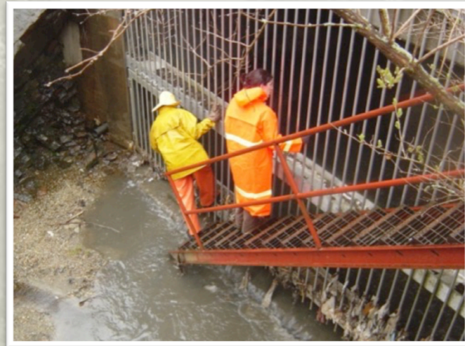
CSO 36, West Side Interceptor Discharge to Fore River Estuary via lower Capisic Brook “Gorilla Cage”
