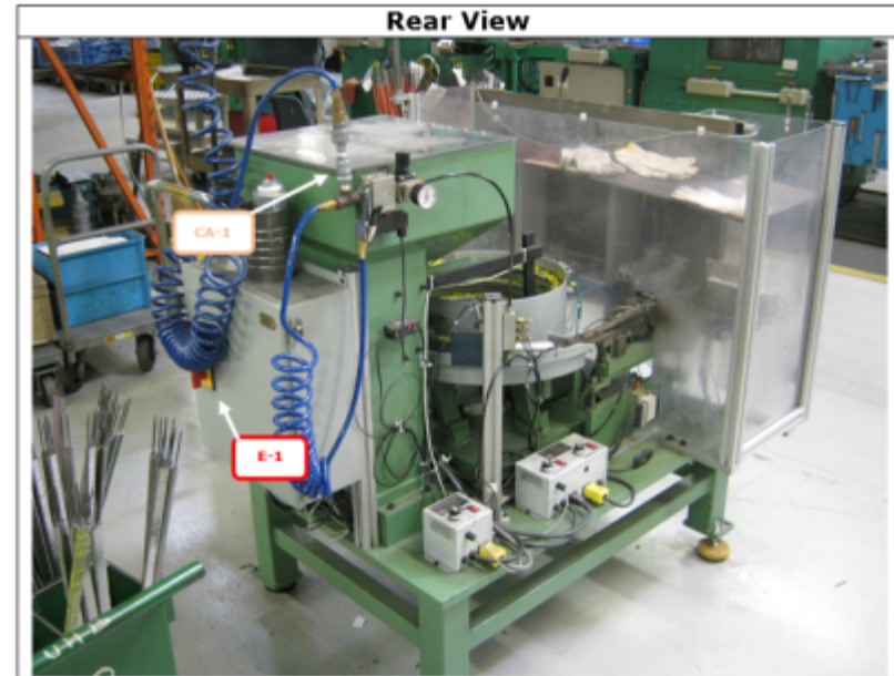
(4) Picture for reference purposes of representing general energy isolation locations for multiple similar machines and may not accurately depict each of the machines listed above. When in doubt, the person performing the lockout should confirm the energy isolation device location and verify proper isolation using the steps in this procedure.
