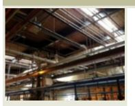
Grinder and Centrifuge Feed Pump Installed Between Press Feed Pumps and Piping
