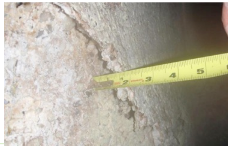
Junction (Home Plate) Chamber Walls
