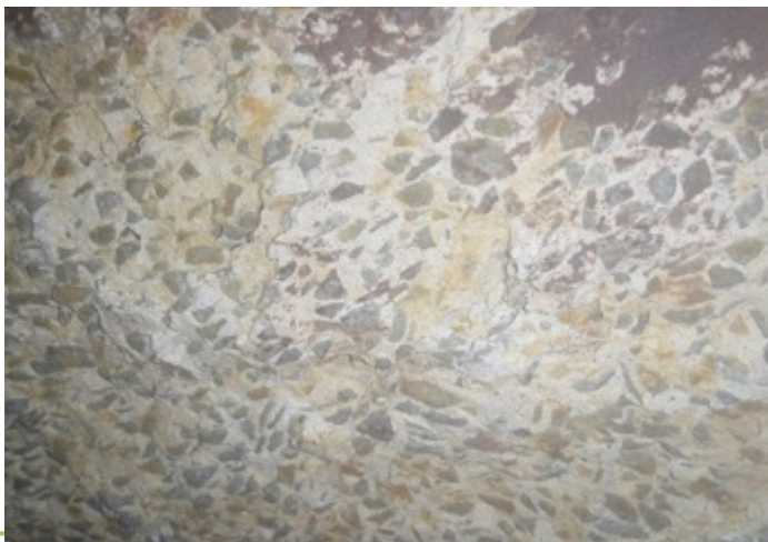
Transition Chamber Wall
