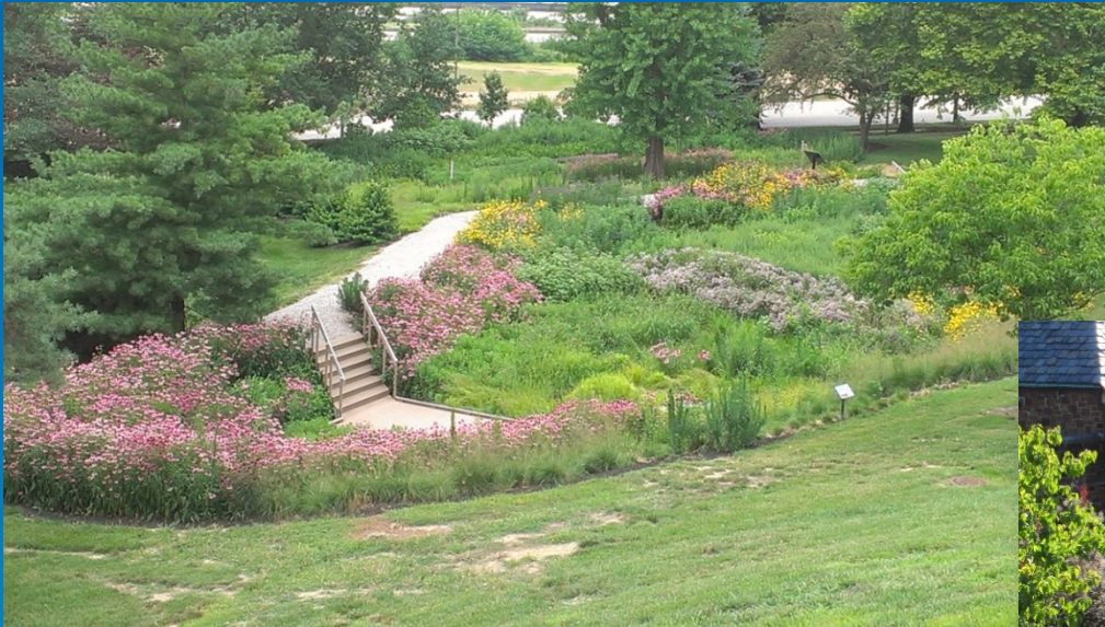
CSTCC Biodetention Basin after 4 years Good condition & well maintained July 2014 R. Mirizzi photo
