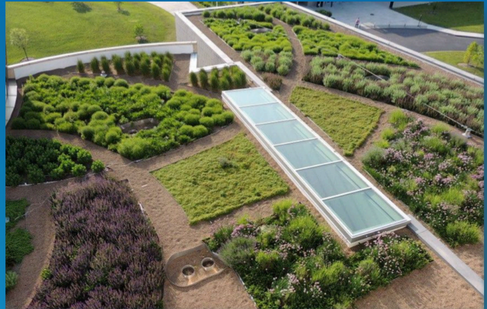
NKU Green Roof July 2014
