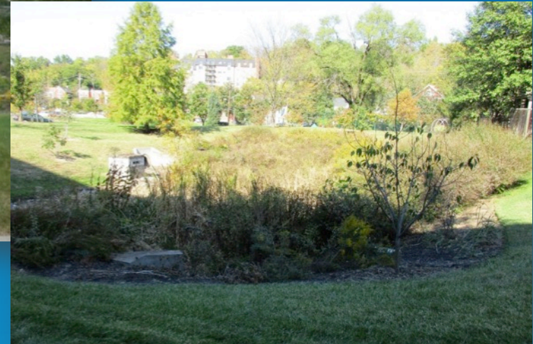
CSTCC Basin Retrofit at 4 years After first freeze – good condition October 2015
