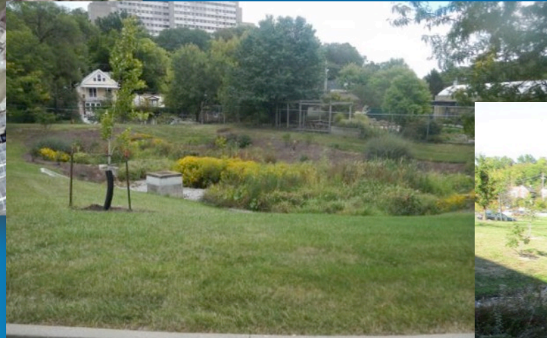
CSTCC Bioretention Basin Retrofits at after 2 years – Good condition September 2013
