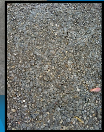
Clark Montessori High School Pervious Concrete Parking Lot May 2013
