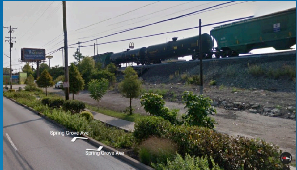
Spring Grove Avenue Bioswale Good condition - Healthy plants, well maintained 2015 Google Earth Street View Photo
