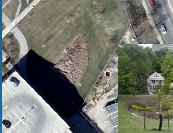
CSTCC Detention Basin – next to Parking Lots – 2007 aerial
