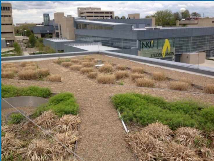
NKU Green Roof after 5 years Colder winter than normal March 2014
