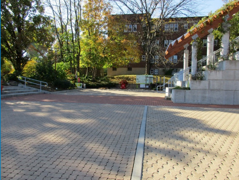
Civic Garden Center – 4 years later Permeable Paving Areas October 2015 K. Couch Photo
