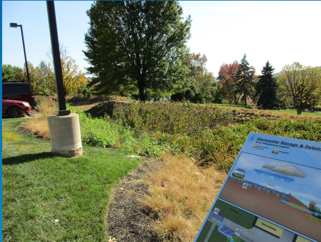
CSTCC Biodetention Basin by Parking Lot – Built in 2010 Five years later - After freeze: Good condition & well maintained October 2015 K. Couch photos
