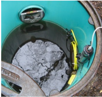
Off-the-Shelf Weirs, Flumes, and Loggers
