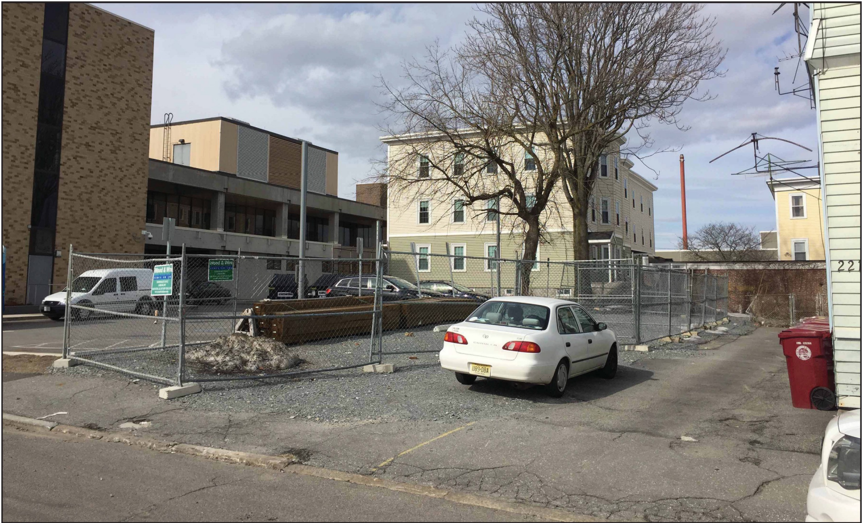
Decatur Way Arbor Structure- Existing Condition Lowell, Massachusetts
