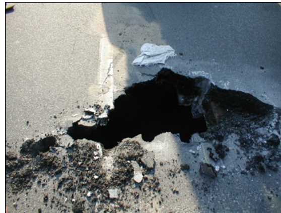
Sewer collapse at crown of pipe
