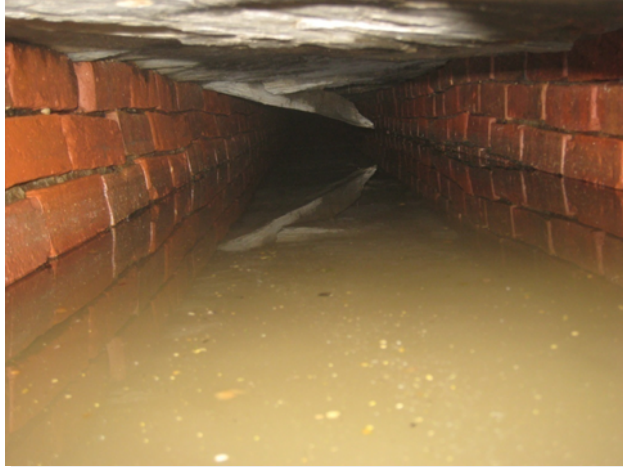
Slate collapse into sewer
