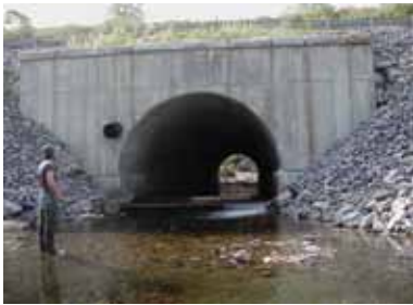
Culvert with perched outlet on Broad Brook
