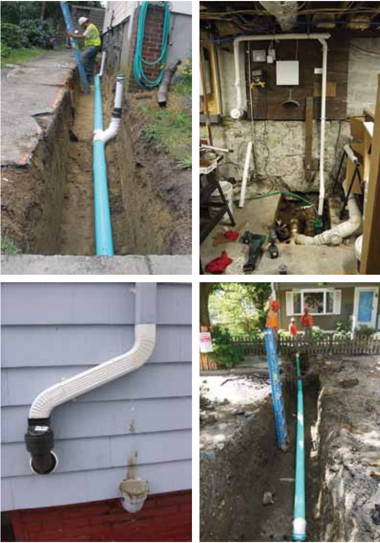
Example of private property inflow removal work being performed in the Huron A, Huron B, and Concord Avenue areas
