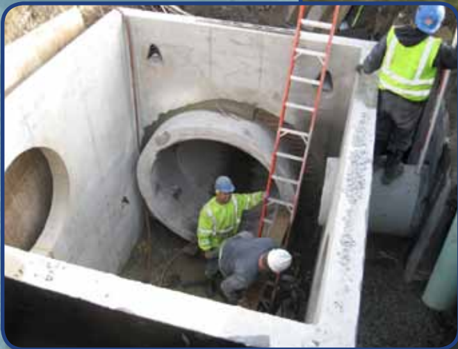
New Drain Manhole Construction – Reserved Channel Sewer Separation Project, Boston, MA
