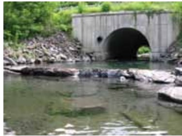
Rock sill constructed to raise outlet pool on Broad Brook
