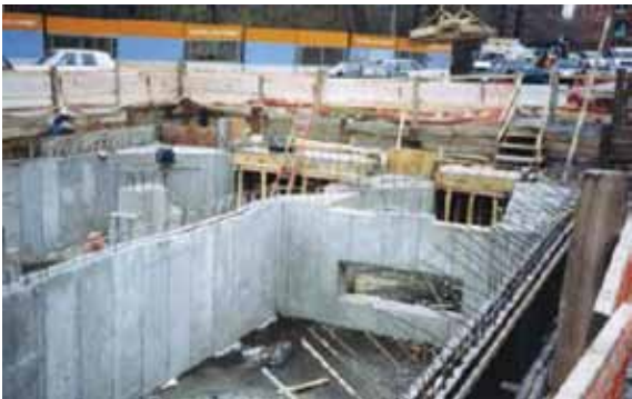
Photo 3. Construction of one of the stormwater flush vaults on Fresh Pond Parkway
