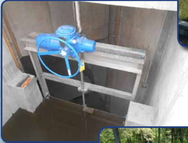
Automated Weir Gate Construction at Combined Sewer Overflow Regulator – Alewife Reservation, Cambridge, MA
