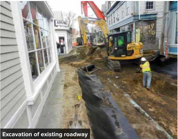
Excavation and stone bed
