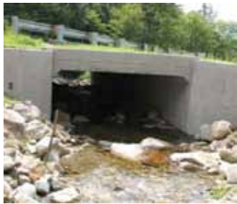
Replacement concrete box culvert with natural substrate
