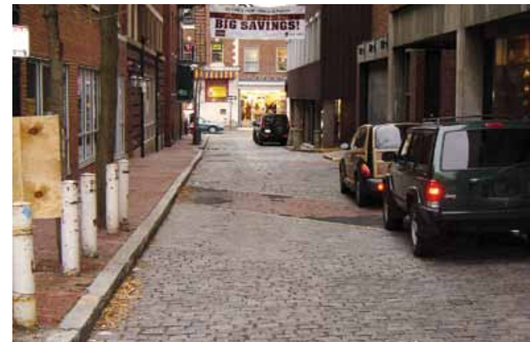
Engineered surface flow channel along Palmer Street near Harvard Square
