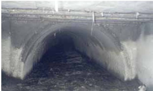
Photo 2. Sediment accumulation in the Wheeler Street conduit
