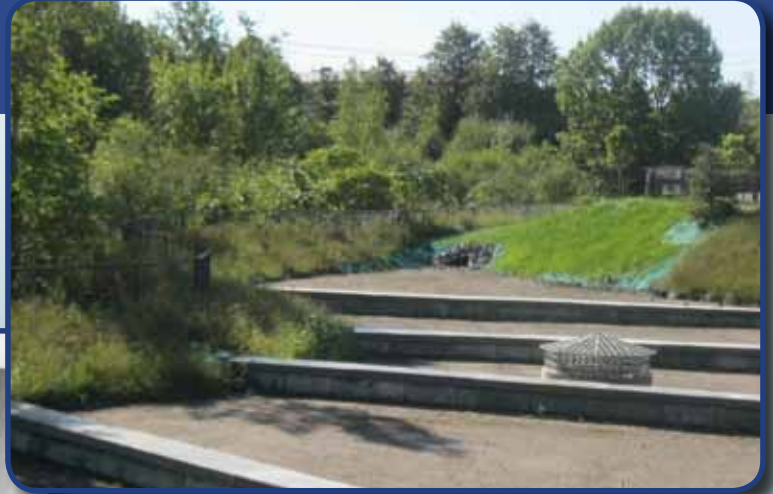
Underdrained Soil Filter Stormwater Treatment System – Long Creek Restoration Project, South Portland, ME
