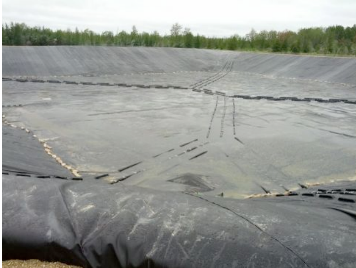
Lined & Covered Storage Lagoons
