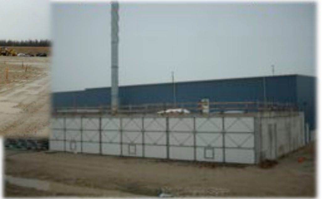
Rear of OMRC – biofilter system
