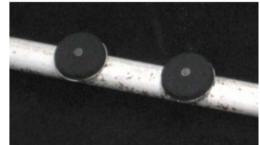
Ceramic Dome Diffusers at Coney Island WWTP
