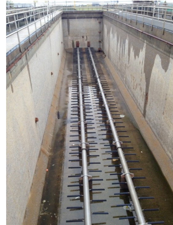
Coarse Bubble Tube Diffusers at Rockaway WWTP
